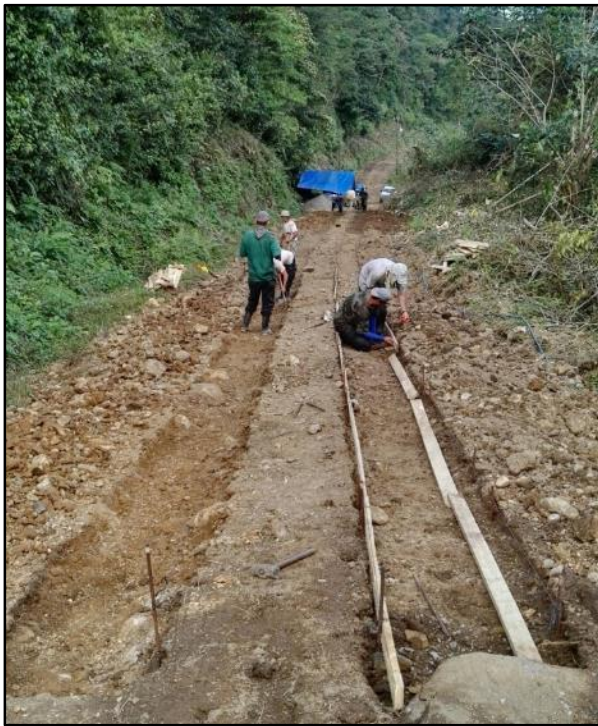
Repairs on the road to Pocosol Station
